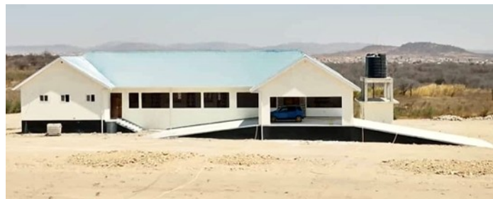
Selemani's crew finished the Outpatient building in record time. Let's help get it ready to open!
