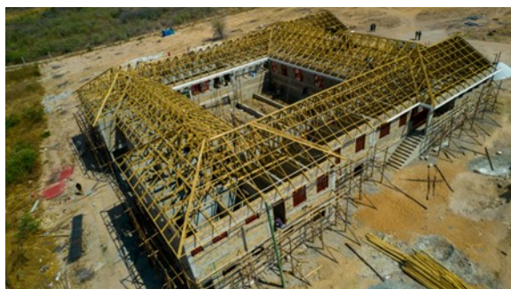
This birds-eye view from July shows the enclosed courtyard waiting area
