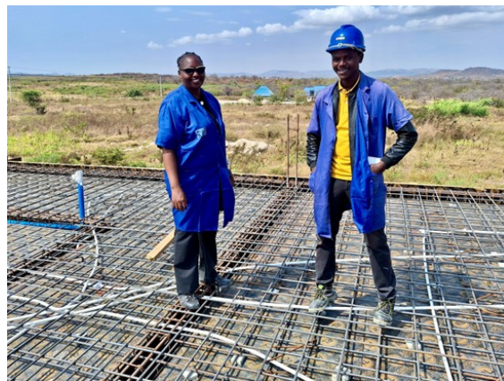
Nurse Miriam and foreman Richie stand on steel reinforcing bars for what will be the concrete second floor of the outpatient building.
