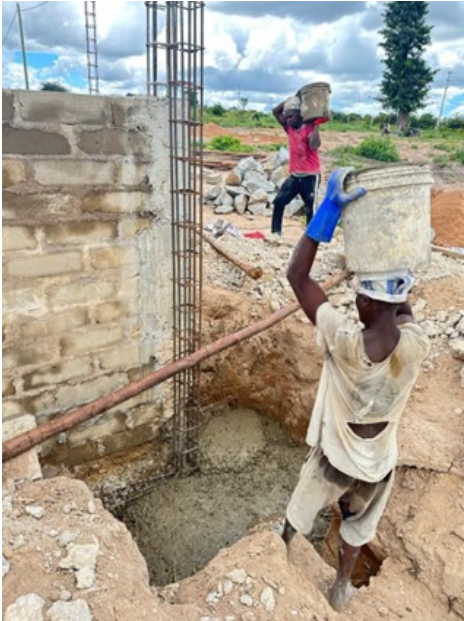
Workers carrying buckets of concrete for the foundation
